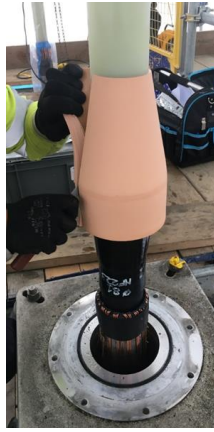
Removal of stress cone, including cable inspection
