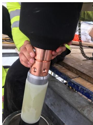
Installing termination on prepared cable end
