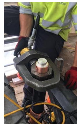
Installing connector / plugset
