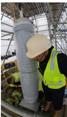
Installing termination on prepared cable end
